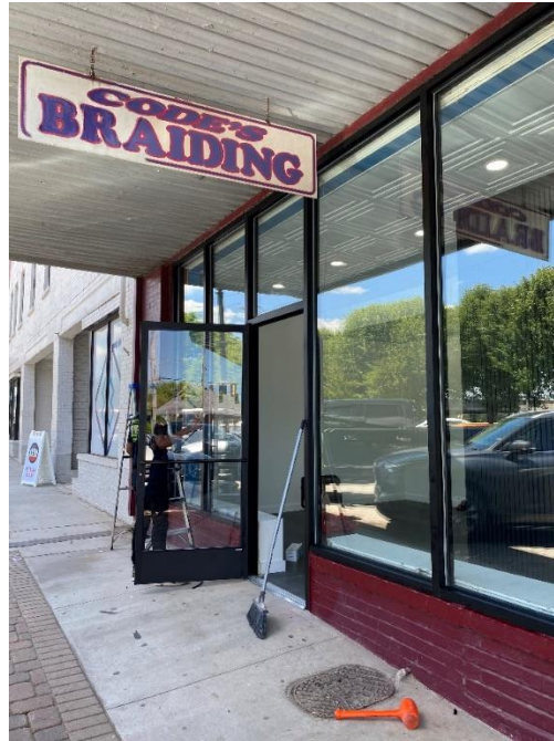
Code's Braiding business improvement, received new windows at 3753 Main St.
